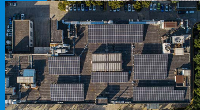
The solar power system installed in our Shanghai, China, manufacturing plant has an annual carbon offset of 245 metric tons.
